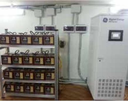
In addition, the Trojan 22-AGM incorporates a computer-generated grid design that is optimized for high-power density, while its low internal resistance provides a higher discharge current and higher charging efficiency. The low calcium grid alloy reduces gas emissions and a flame arresting, one-way pressure relief vent prevents buildup of excessive pressure. The Trojan 22-AGM also is certified as a Sealed/Non-spillable (UN2800) battery approved for air, sea and ground transportation.
